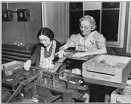
Clip spring and body assembly for .30 caliber cartridges
